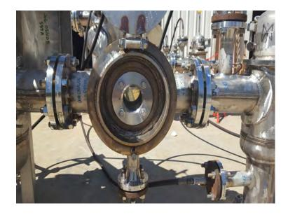
Visual samples not enough? You can take physical samples with the Lookbox. We can modify or add a top access lide to your Sultrap<sup>™</sup>, Sulview sightport, or flange for physical inspetion and examination of the contents.
